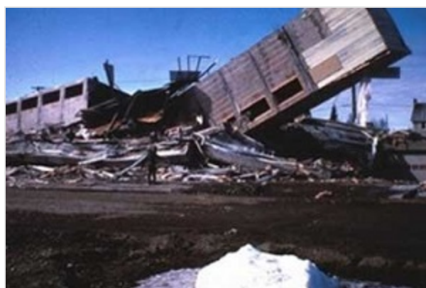
Collapse of the newly completed Four Seasons Apartment Building in Anchorage during the 1964 earthquake
